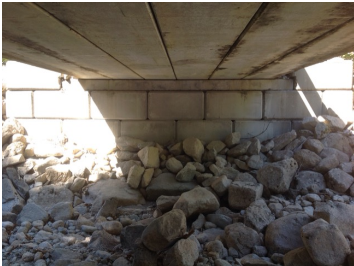
Right Bank Abutment when facing downstream
