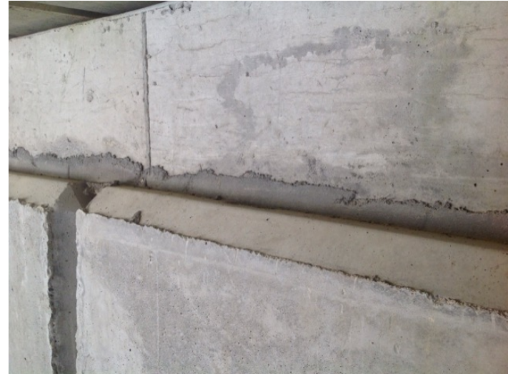
concrete cap grouted to lock blocks
