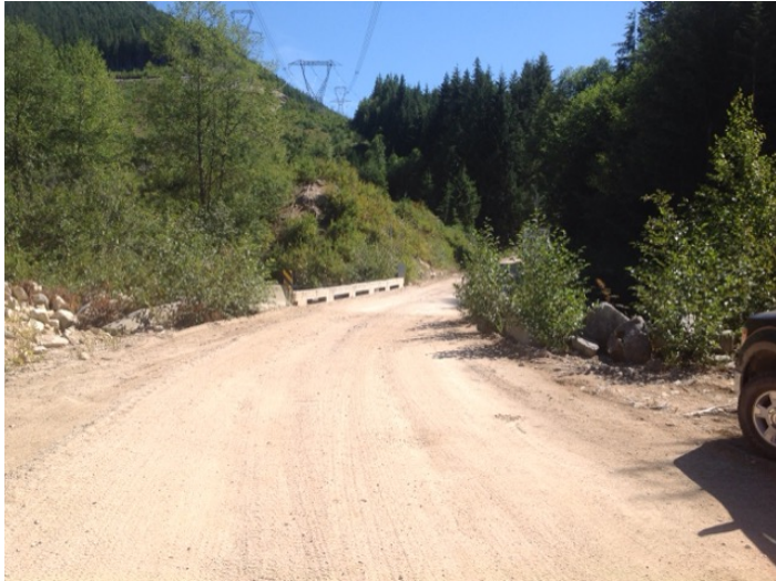
Approach from Right Bank when facing downstream
