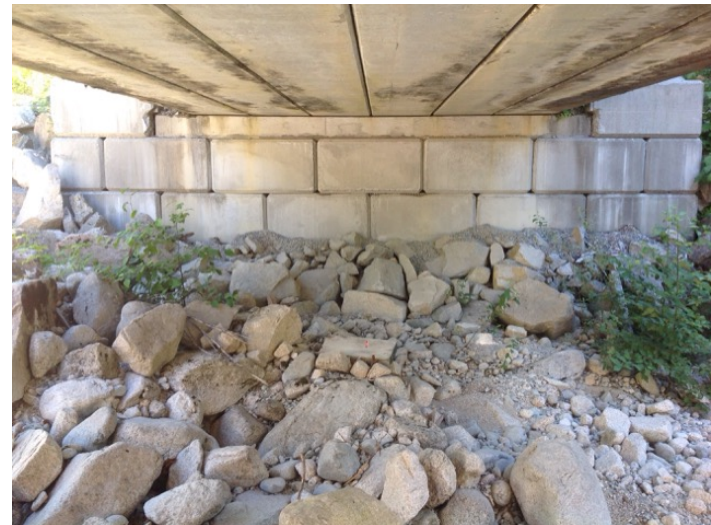
Left Bank Abutment when facing downstream
